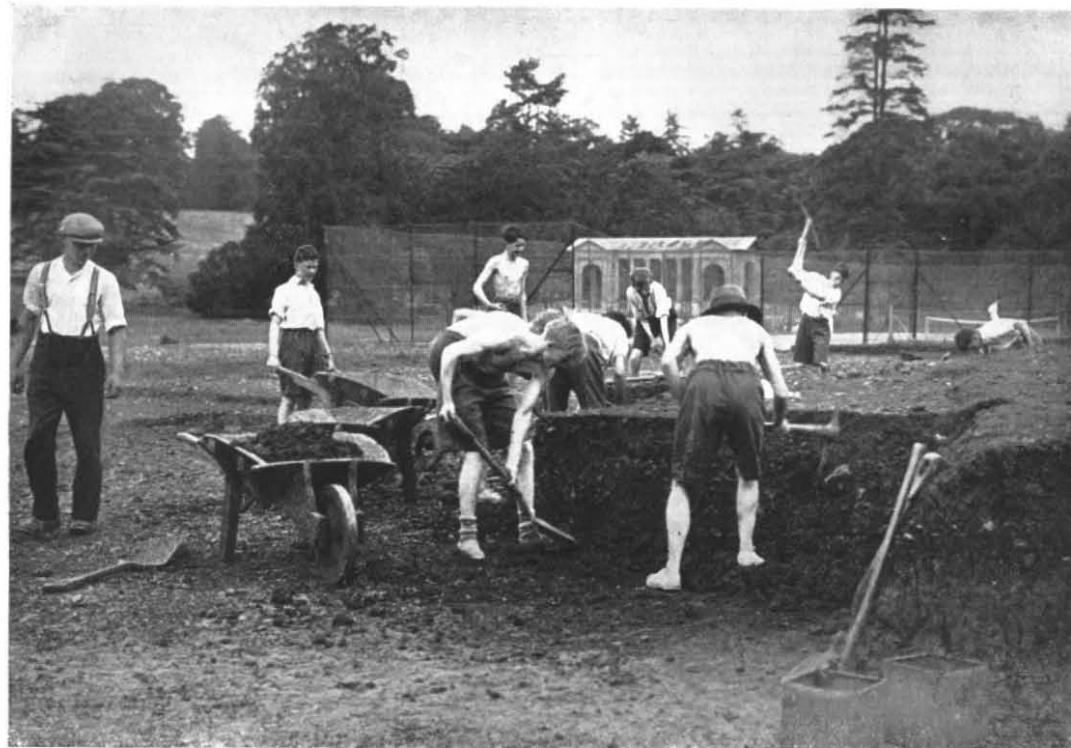
WORK ON THE PALLADIAN TENNIS COURTS.
